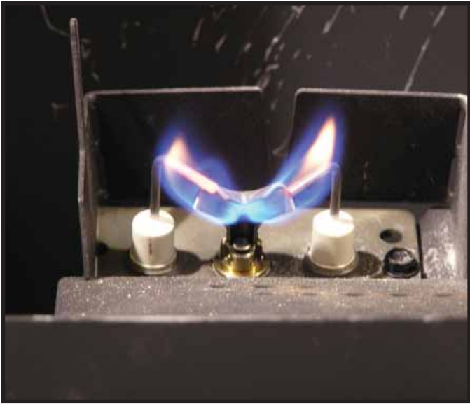
Figure 3.1 IPI Pilot Flame Patterns
